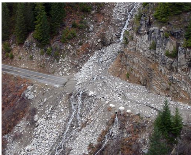
Figure 11: Example of a landslide impacting roadway in Cascadia
